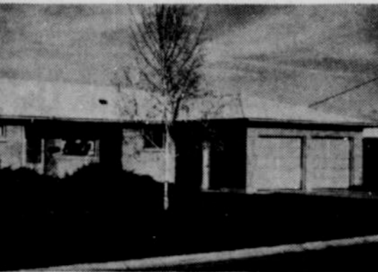
MORE THAN 1100 existing homes have been changed to electric heat, including that of the Masons at 4020 Hillcrest Drive in Boise.
