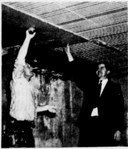
ABOVE: With radiant ceiling cable heat, wires are stapled to the ceiling and covered over. There are no moving parts.
