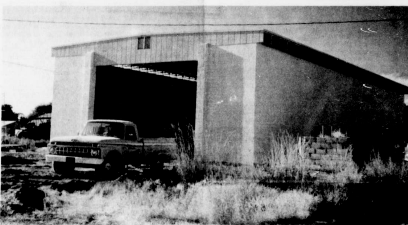
THIS IS THE SOUTH END OF A NEW BUILDING ON EMISON street in Nyssa, between 8th and 9th streets. While not yet fully completed, it will house the operations of Dority Bee Boards, owned by John Dority. He has been drilling bee boards as the home for leaf-cutter bees. These are the smaller type pollinators that are so useful in the western area due to their making their nests in small holes in old boards where they deposit the larvae for a replacement for themselves the next season. Dority has had a board-drilling operation in a small
