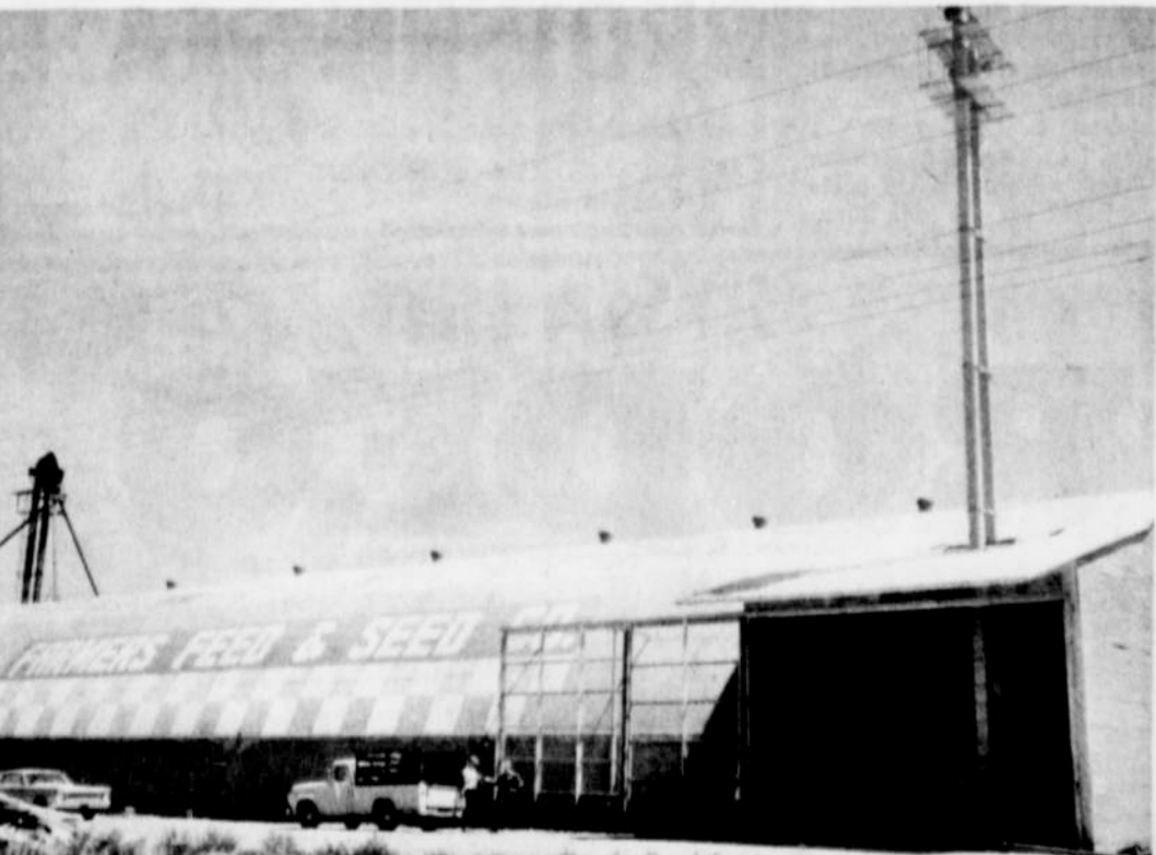
The high warehouse building isn't new but the 75 foot high elevator at the right end of the structure is. It was recently completed by Parma Water Lifter company and Holcomb Construction to speed up unloading of grain at harvest time. This is the only warehouse in the Lower Treasure Valley having an elevator to move wheat and another to move barley
