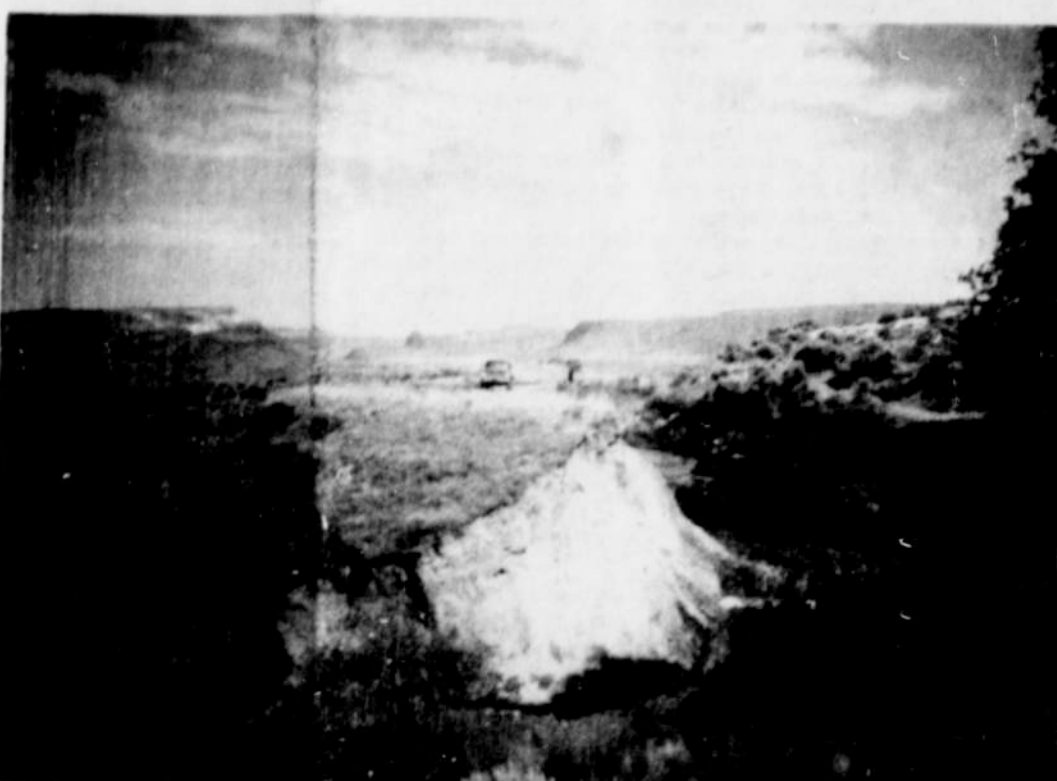
Pictured above is the break in the Kingman lateral that occurred about 7:30 a. m. July 4th near the Mendiola ranch 6 miles west of Adrian. The vehicle in the center is immediately above the west bank of the old channel. Left center shows water where the break occurred and the
