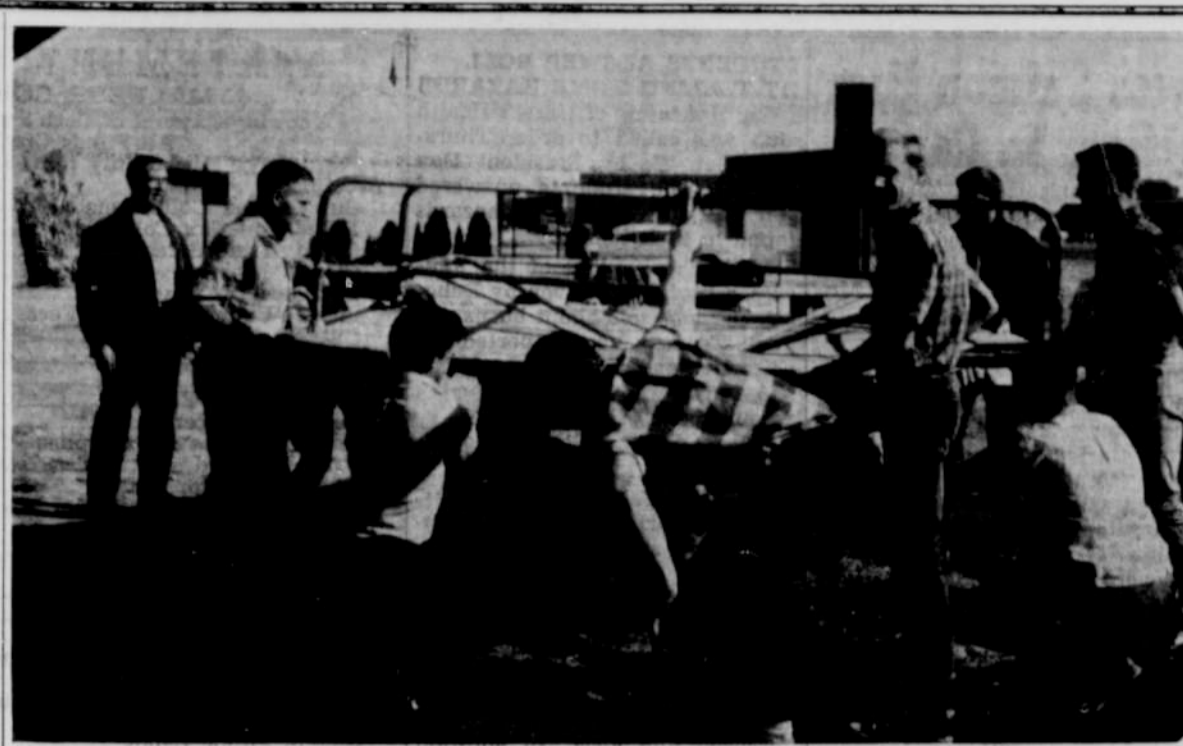
LATEST PROJECT of the NHS vocational agriculture III class was a sidewalk encircling the merry-go-round on the primary school campus. Work done by the students included everything from transit operation to cement finishing. Pictured (left to right) are Adviser Stanley Sisson, Eldon Widmer, Marcelino Soliz, Connell Petterson, Fred Esplin, Jim Farmer, Charles Belveal, Lynn Draper, LaVern Widmer. Other participants, not pictured, were Jack Wilson, Royal Snyder, Karl Smith, Manuel Silva, Fred Schilling, Clinton Robbins, Delmar Phillips, Roy Carroll and Roger Nakashima.
