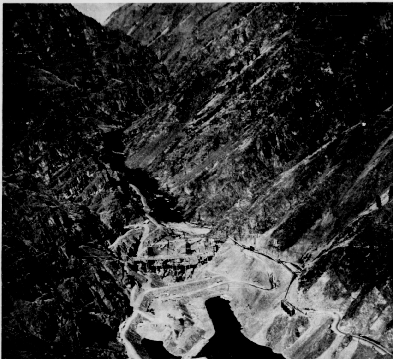
AERIAL VIEW LOOKING DOWNSTREAM, with Oregon at left and Idaho at right, shows narrow, mountain-walled gorge where Idaho Power company is building Hells Canyon dam for completion in 1968. At center, beyond temporary upstream cofferdam that turns the Snake river into diversion tunnel, is 200-foot-high steel trestle from which three whirley cranes are placing concrete
