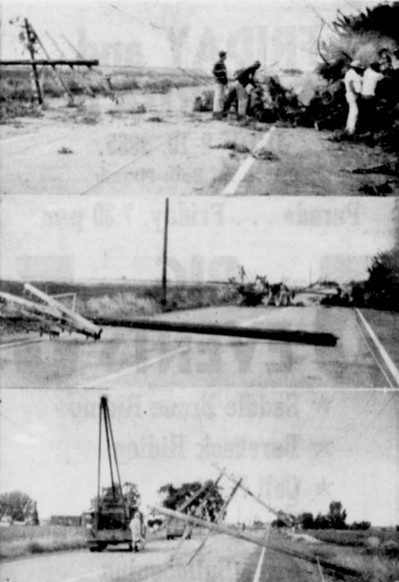
THESE PHOTOS SHOW THREE of 28 telephone poles that toppled like lined-up dominoes during a freak windstorm which hit a section just north of Nyssa late Saturday afternoon. The pictures were taken at various locations on highway 20-26, several hours after the damage was done. Workmen from Malheur Home Telephone company's service department were already working to clear the highway which was blocked for a two-mile stretch until Sunday night and then again on Monday while the crews continued to work. Service was partially restored at approximately 11:30 on the night of the storm, according to a telephone company employee, and at 6 p.m. Tuesday restoration was about 70 percent complete. A downed tree in front of the rural home of Mrs. Tom Jones apparently started the chain reaction and boosted by the strong wind, the poles snapped off one by one. They were not uprooted. Known to be traveling on the highway when the storm struck were Mrs. John Olsen; her mother, Mrs. Ada Garrison; her daughter, Trudy Olsen and Mary Danford in one vehicle and Miss Karma Kesler in another. They managed to turn their cars around and scamper out of the area, as the poles fell behind them. Miss Kesler told a Journal reporter that if anyone ever turned around on a dime and headed the other way, it was she that afternoon.—Staff Photos.
