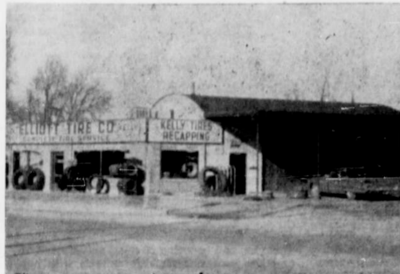
THIS IS THE ELLIOTT TIRE FIRM, owned and operated by Mr. and Mrs. Bob Elliott who came to Nyssa early in 1960 from Portland where they owned a similar business. Early in June that year the structure was completed, the Elliots began their tire recapping and repair business and on June 18 held their grand opening event at 204 North Main street.
