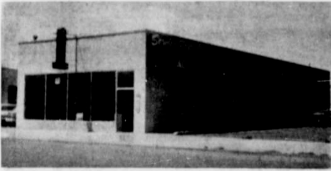
CONSTRUCTION of this building was begun early in October 1960 by Lee Cables of Ontario. It is the home of Service Parts company, an automotive store, located at 17 North Fourth street. The structure and a paved parking lot were completed early in December that year and the business was moved from the Peterson Furniture building at 223 Main street.
