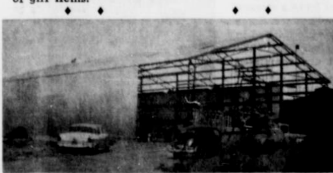
THIS IS COMINCO's fertilizer storage warehouse when it was under construction in August 1961. It is located on the Union Pacific railroad spur near the intersection of South First street and King avenue, and is a distribution center for Elephant Brand products. The all-steel structure has metal roof and walls with reinforced concrete foundation and floor. The interior measures 58 x 99 feet, with 18-foot walls.
