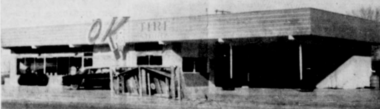
ONE OF THE MORE RECENT ADDITIONS to the commercial firms of Nyssa is Ray Tarter's O.K. Tire retail store. The structure was completed and was opened for business around mid-
