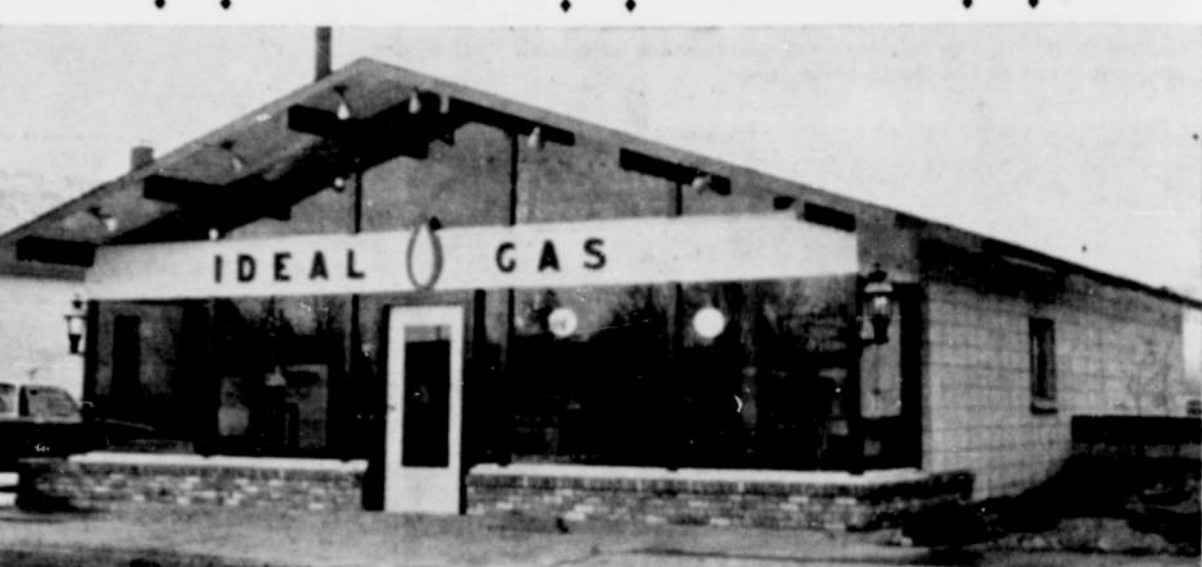
OPEN HOUSE was held Dec. 17, 1963, at the Ideal Gas and Appliance firm, owned by Wilton and Margery Jackson. The new structure replaced the old one which was destroyed by fire on Aug. 14 that year. The building is constructed of brick and concrete block and the front is glass-paneled from foundation to roof. It is located at 14 North First street.
