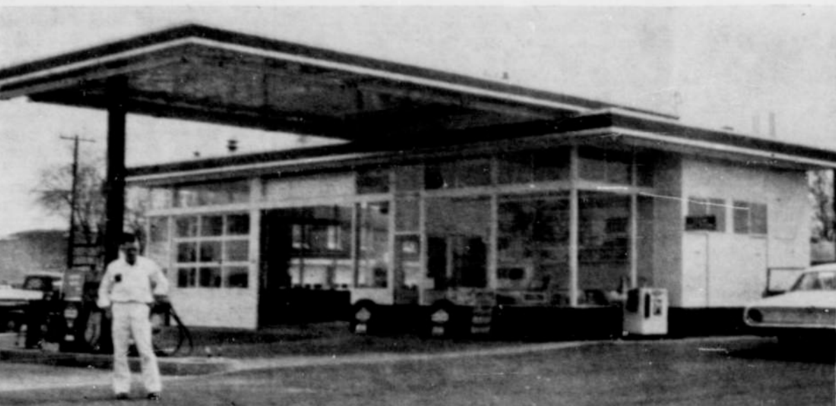
ANOTHER RECENT ADDITION of Nyssa business firms is the all-new Chevron station located at Third and Main streets, former site of the old Signal station. Construction was completed early in 1965 and the grand opening event was held April 10 this year. Manager Harold Kassman and his family came to the Nyssa area from Sprague, Wash.
