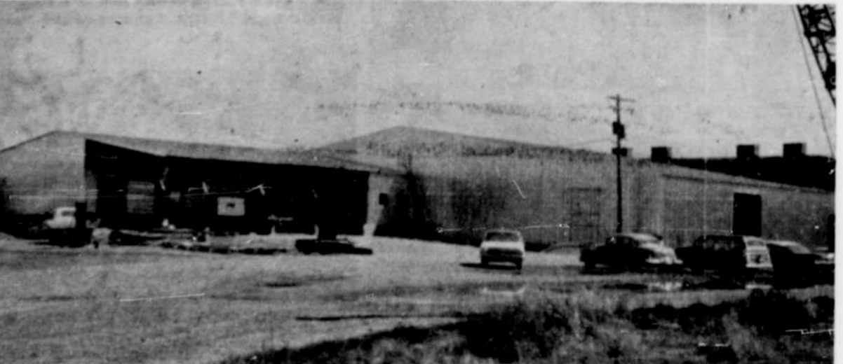
CONSTRUCTION on the J. R. Simplot building 20,500-square-foot structure houses a 52- x 78-foot packing shed, offices and a 96 x 150 produce storage area. It is located at Walnut and the UP railroad tracks.
