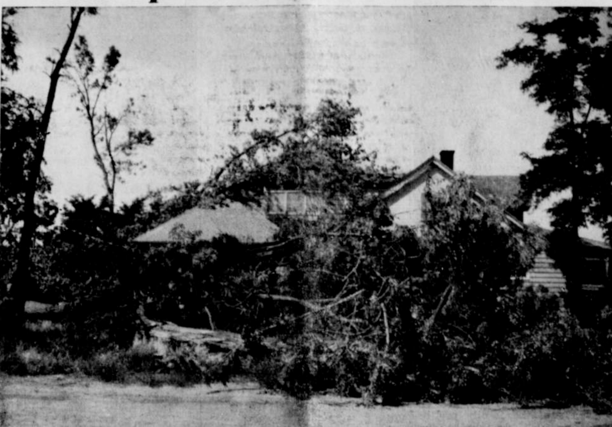
THIS IS THE SOUTH SIDE of the John Stringer home, southwest of Nyssa, nearly obscured by uprooted trees after the high windstorm on the evening of July 29. Some of the trees fell directly on the structure. At the time this Journal photo
