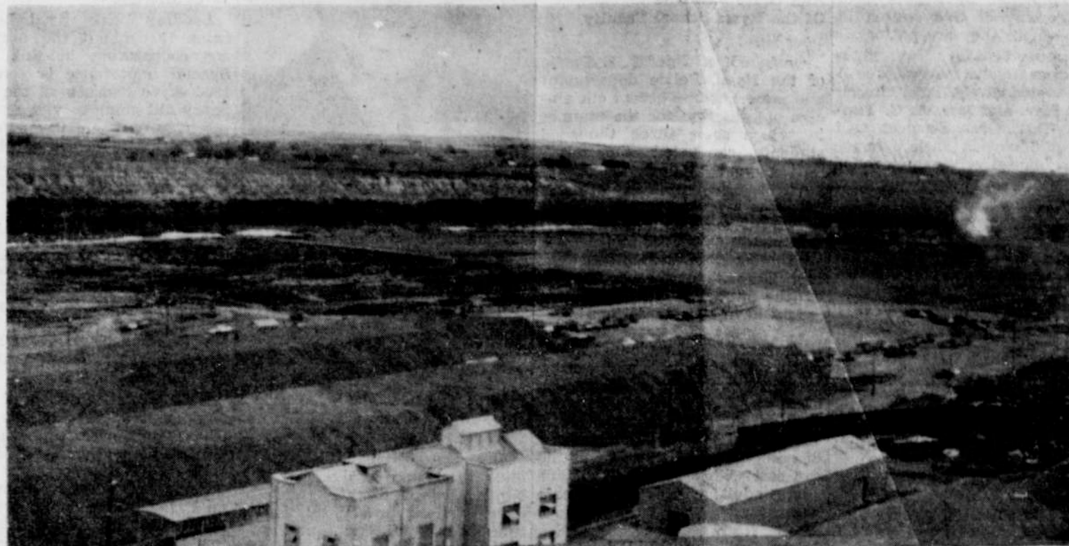
THE TWO BEET PILES (left foreground) don't look very large from the top of the 160-foot-high silos at Nyssa's Amalgamated Sugar factory, but they are 800 feet long, 140 feet wide at the base, 80 at the top and 22 feet high. There is another the same size to the left of these and the fourth pile was being started when a Journal photographer took this picture Monday afternoon.
