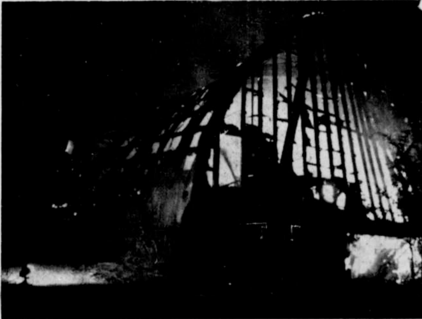
THIS PHOTO was taken by a Journal photographer just before collapse of the framework of the Royal Produce warehouse which was destroyed Saturday night by fire. The structure was owned by the Sadamori and Hirai brothers.
