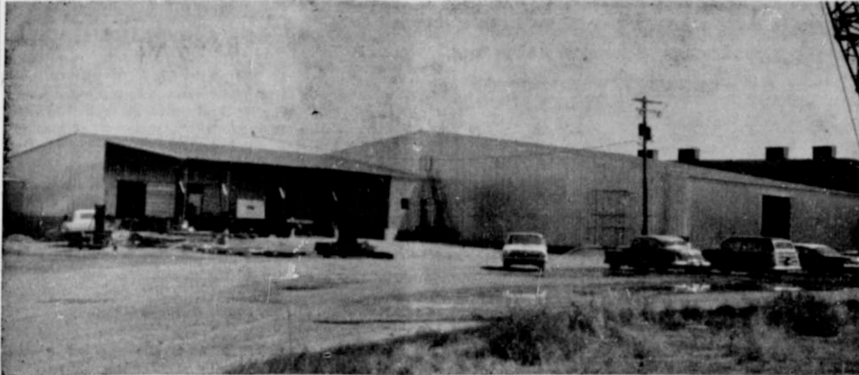
THE J. R. SIMPLOT PACKING SHED pictured above will be entirely completed in the near future. The 20,500-square-foot Garceau steel structure replaces the one destroyed by fire on March 25 this year. The building houses a 52 x 78-foot packing shed area and a 96 x 150-foot onion storage space. Construction started in mid-June. The plant, under management of Mas Yamashita, has been in operation for the past two weeks and potatoes are being processed. Work on the office is virtually completed and personnel has moved in. —Staff Photo.
