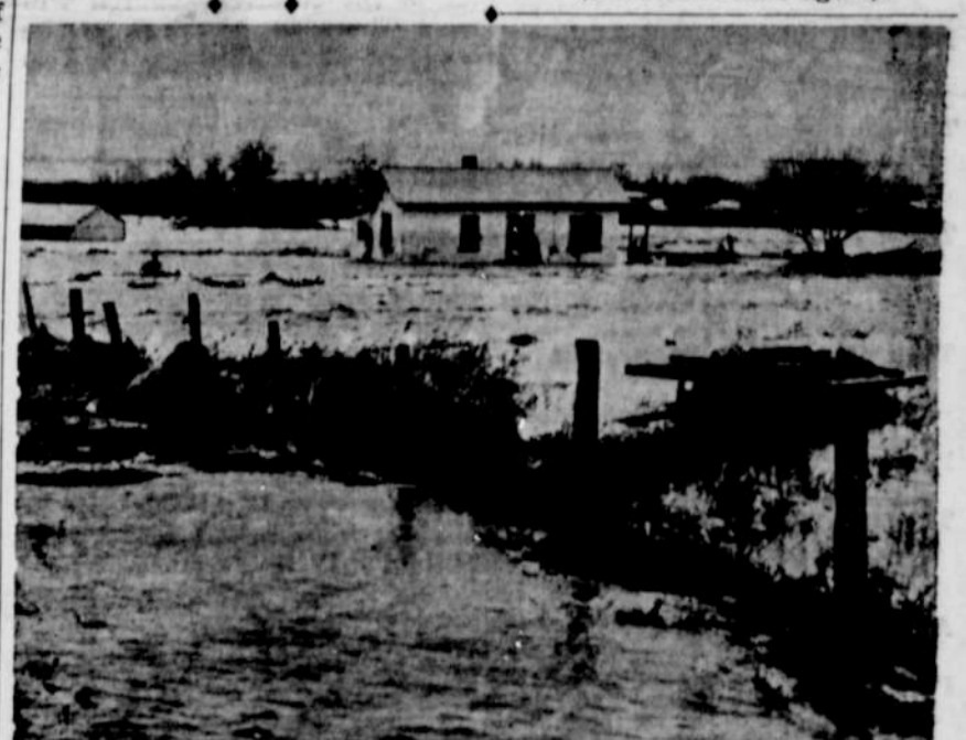
SCENE AT THE GEORGE ROLAND HOME near Homedale when little Succor Creek became a raging torrent Jan. 31 and Feb. 1 following a warm rain and wind melting snow at upper elevations. The seven members of the family were trapped in the attic of the home until rescued by a National Guard tank driven by Sgt. Dean Huffman about 6 a.m. on Feb. 1. (Photo courtesy of the Owyhee Chronicle.)
