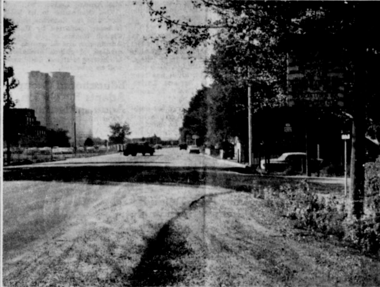
THIS PHOTO was taken Monday on Nyssa's East Main street, looking west. It reveals the vast difference in the width of the highway on opposite sides of the intersection. Curbing, guttering and drains were completed by the city prior to the highway department's paving work past the sugar factory, which was completed before the beet trucks began to roll on Oct. 2. Remainder of the paving project to the Snake river bridge will be done later. To the extreme left in the photo may be seen a portion of the White Satin sugar factory and storage silos. A beet truck has just left the dump yards to return to the field for another load of sugar beets. On the far right is the Nyssa service clubs sign near the intersection of East Main and East Third streets. —Staff Photo.
