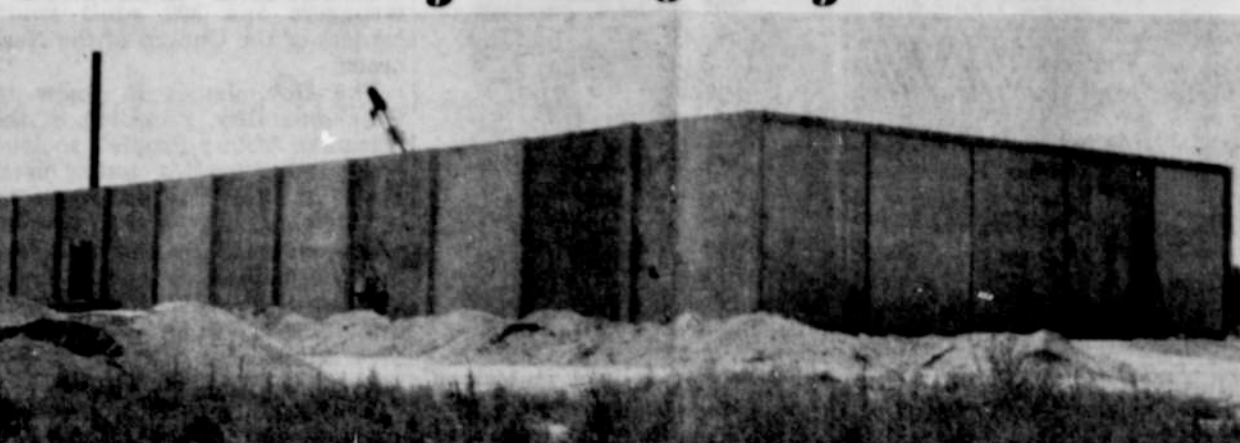
THIS STRUCTURE is being added to the present Idaho Canning company plant in Nyssa. The 90-by-240-foot building of concrete and reinforced steel is being built on to the north side of the factory, parallel to the railroad tracks, and according to President Fred Moss, will double present storage. Completion date is set around Aug. 1. Photo was taken Monday by a Journal photographer.
