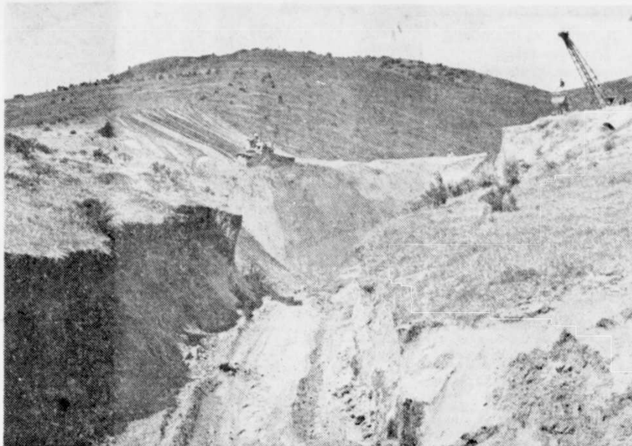
A WASHOUT on a main lateral of the Owyhee ditch near Malheur Butte early Friday, April 27, brought most of the personnel and their equipment
