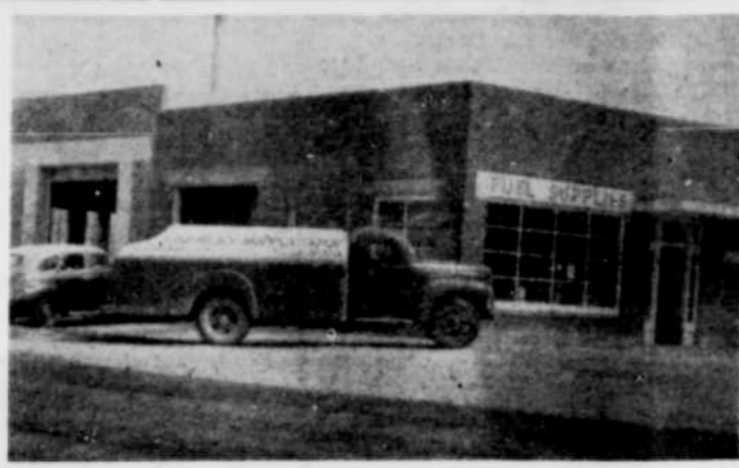
The Farmers Supply co-operative building, with the new addition recently completed, is shown as it stands at First street and Bowers avenue. The front of the addition is of brick and the other three walls are concrete.
