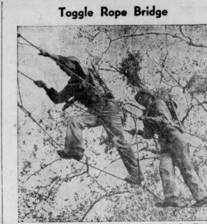
U. S. Marine Corps Photo Quickly strung across otherwise impassable gulches and streams, this bridge is included among the important equipment carried ashore by U. S. Marine Raiders. The three Leathernecks are mastering its mysteries at Camp Pendleton, Calif.
