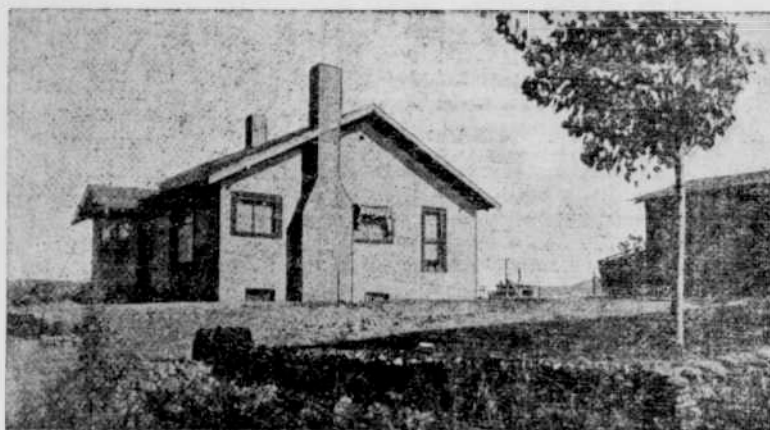
New Home on Vale Project
