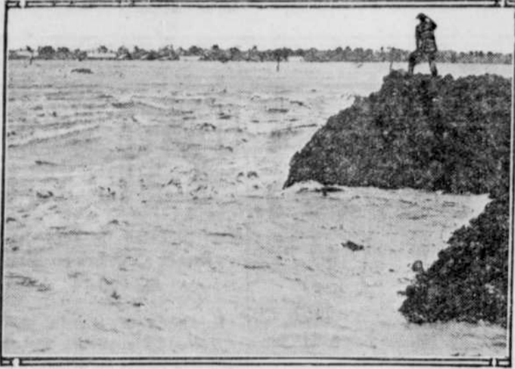
Flood Waters Raging Through a Break in a Mississippi Levee.
