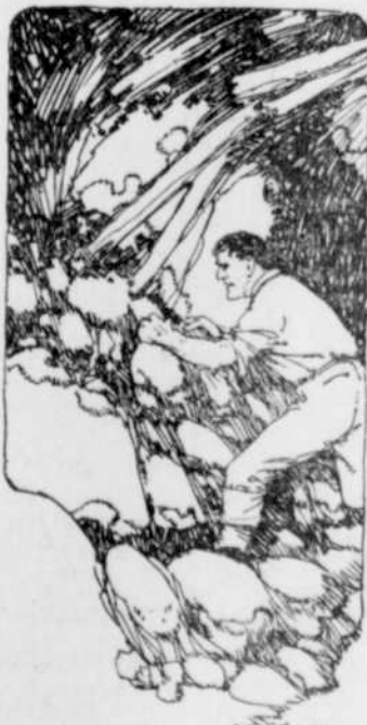
But Even in His Delirious Condition He Stuck to His Work in the Tunnel.
