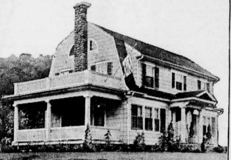
floor plans. However, there are several features of the interior that deserve special mention.
