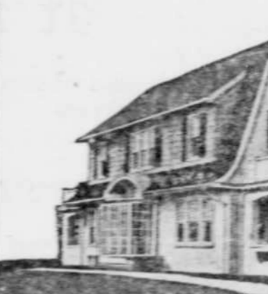
Illustration. In this design the colonial balance is maintained both in the exterior and interior. It will be noted by comparing the exterior view and the floor plan, that the entrance is in the center of the building; that the windows on either side are duplicate, and that there is a similar open porch at either end. This same balance is carried out on the second floor. The gambrel roof, and the long sweep that the roof makes to the second floor sill are graceful. Taken all together this is a mighty handsome home from the exterior.
