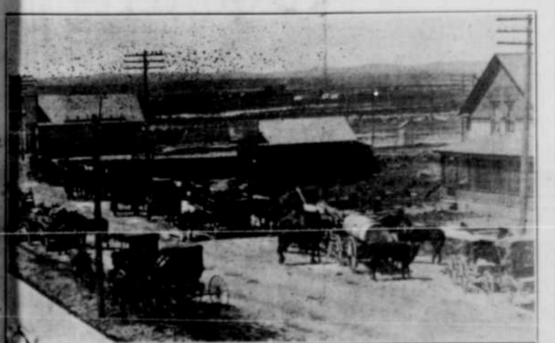
Street scene in Nyssa last Tuesday, showing the railroad grading outfits loaded and starting for the construction camp of the Nyssa-Buhl extension, which is now looking down both ends of the line.
