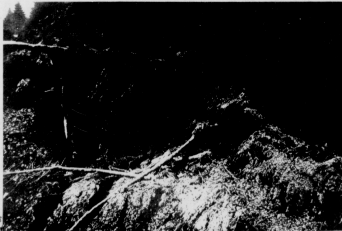
THE SMALLER earth slide that blocked through traffic on the Scappoose-Vernonia highway was only about 50 feet across and some 50-60 feet in depth but it will necessitate extensive repair work before this section of the road is open again.
