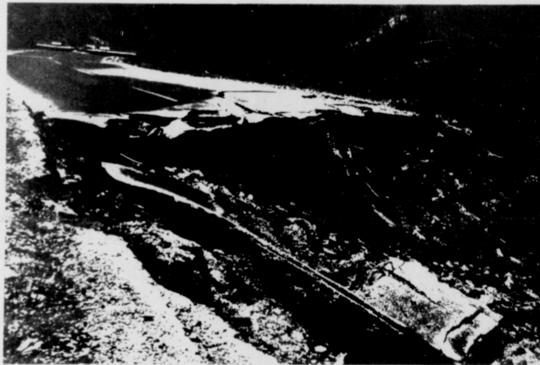
THE SMALLER earth slide that blocked through traffic on the Scappoose-Vernonia highway was only about 50 feet across and some 50-60 feet in depth but it will necessitate extensive repair work before this section of the road is open again.
