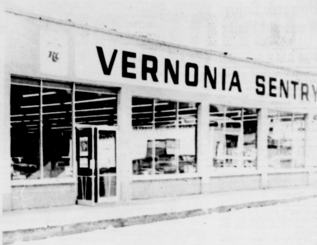
CLIFF'S SENTRY officially became Vernonia Sentry Market last week with the painting of new signs on the building to accompany other remodeling now taking place.
