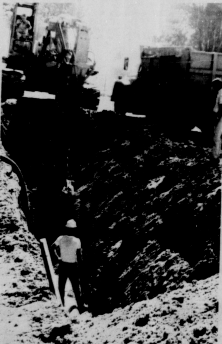
EAST VERNONIA sewer project progresses as pipe-laying crew adds footage to collector system on Knott Street. The recent dry weather has been a boon to the contractor who is hurrying the project through to completion so hook-ups may be made by homeowners prior to winter rains setting in.
