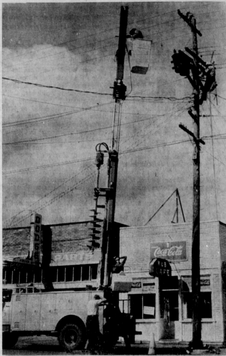
NEW line truck placed in use by West Oregon Electric month and a half ago provides equipment for complete line construction and repair work in one unit. Truck is 2 1/2-ton International with hydraulic winch on boom capable of lifting 9000 pounds and extending to 41-foot height. A nine-foot section at the end of the boom and the bucket is constructed of plastic and is fully insulated. Man in bucket can control action of boom. Earth borer is constructed to bore through rock where necessary and can dig 12-foot deep hole in three minutes in earth. Truck also operates generator to provide power for hand tools. Buck Holsay was in bucket when photo was taken. Tracey Hanson is on pole and Charley Hickman is beside truck.
