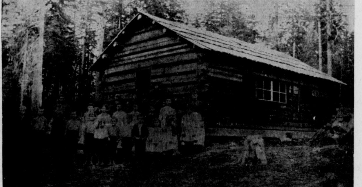
YOUNGSTERS living in Vernonia first went to school in this building, the first school house in town. The structure, built of hewn beams with hand split shakes for roofing in 1889, was located in front of the home now occupied by Mr. and Mrs. J. W. Acaturri. Photo, owned by Bob Spencer, was taken in 1890 and the first teacher was Miss Lovelace. Students included such names as: Gilliam, Mellinger, Emmons, Mills, Peck, Ivy, Lavender, Spencer, Tucker, Parmer, Hosford and Rose.
