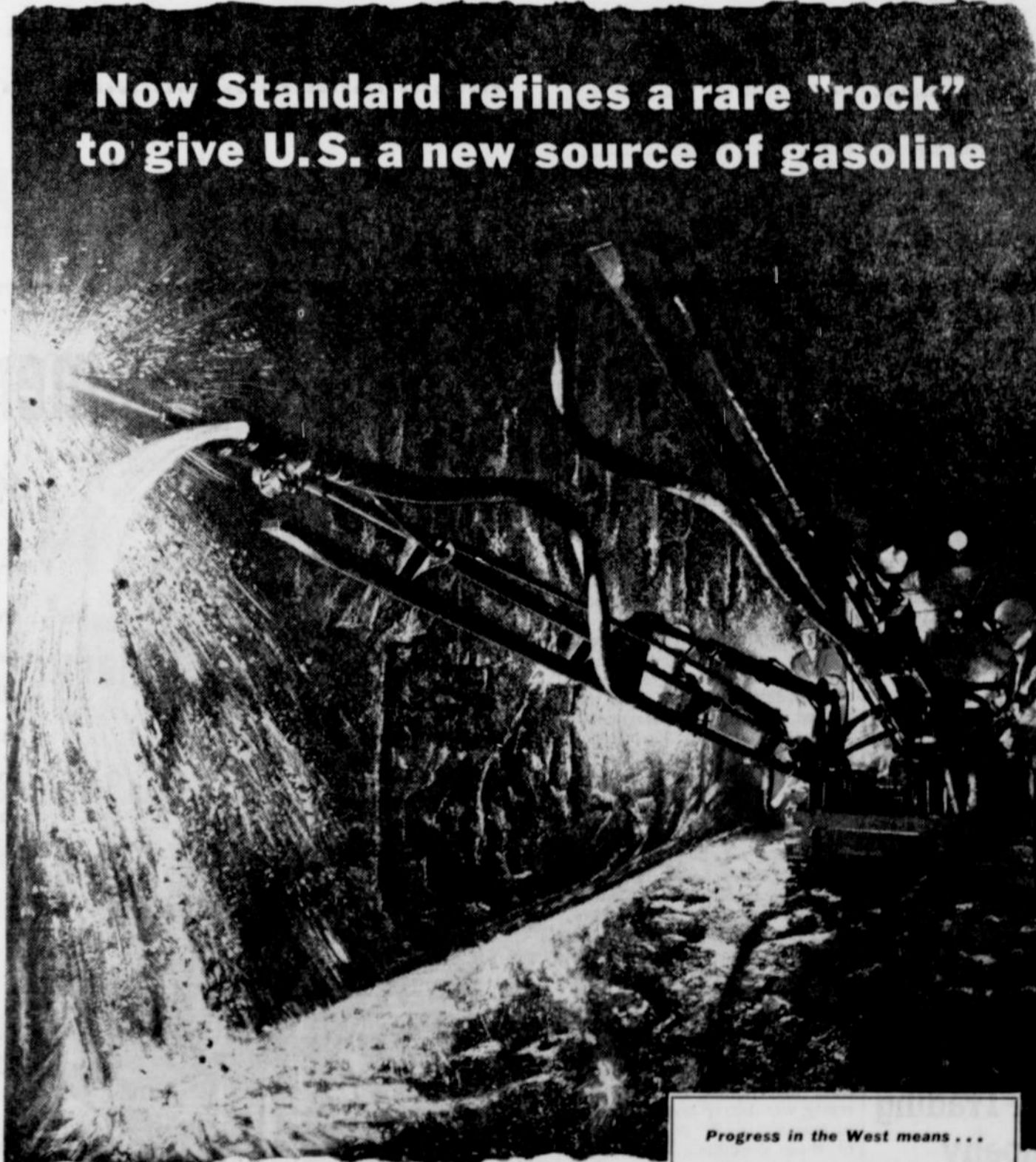
High pressure water jet shatters solid Gilsonite. Flame hose washes particles down mine floor to pipeline.
