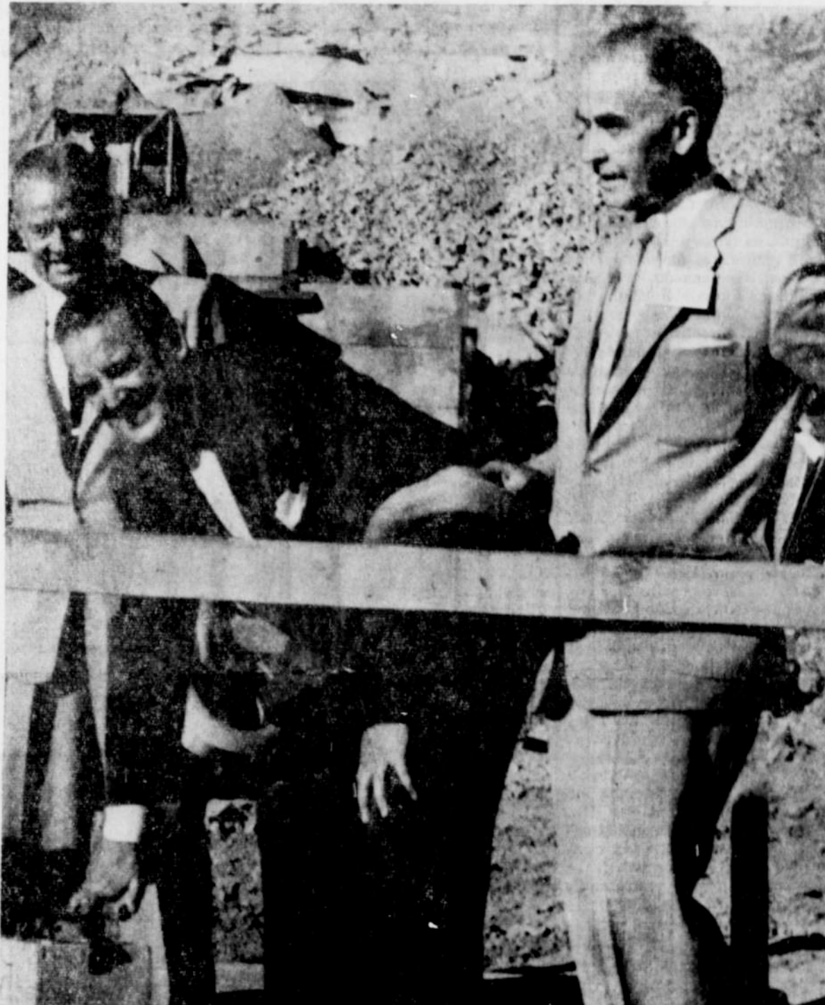
GOVERNOR ROBERT D. HOLMES set off blast last Thursday afternoon in lieu of christening to observe open house at Smithwick Concrete Products aggregate plant at Haydite. At left of Governor Holmes is David C. Duncan, president of Portland chamber and at right, S. Carl Smithwick, head of firm. Open house was attended by many state officials and Vernonia people to observe start of operations at plant.
