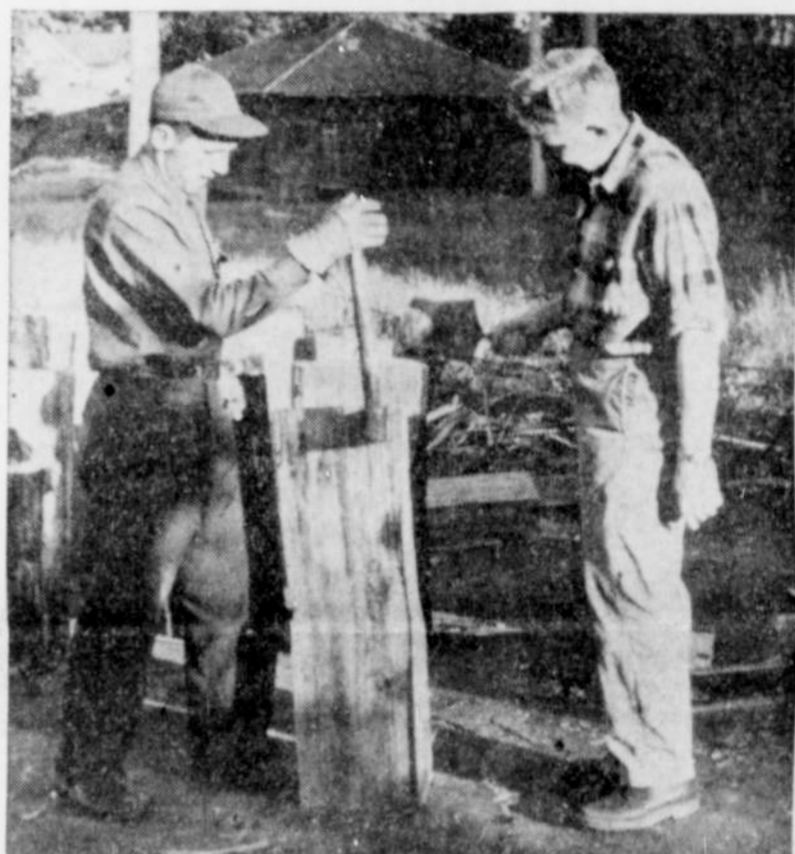
ROOF and part of sides of Lions park project will be finished with shakes being split here by Joe Magoff and Bill Horn. Several other crews of Lions have been busy splitting so sufficient shakes will be available when framing of structure is completed.
