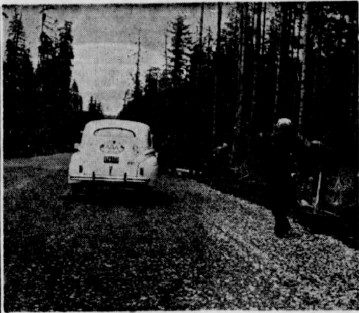
The motorloggers stopped on a graded section of the highway to "kibitz" WPA workers leveling the crushed surfacing rock.
