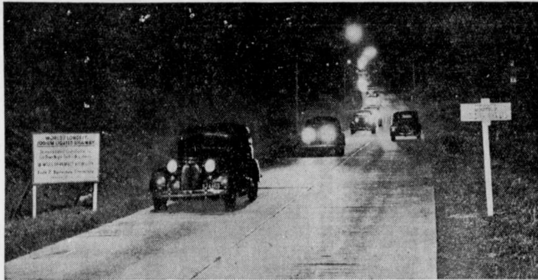
A motorist can see a pedestrian a half mile ahead and a car three-quarters of a mile ahead at night on the illuminated highway between Schenectady and Duquesburg, N. Y. The 18-mile stretch of road is lighted with 390 yellow sodium lights spaced 250 feet apart by engineers of the General Electric company and the American Road Builders' association.
