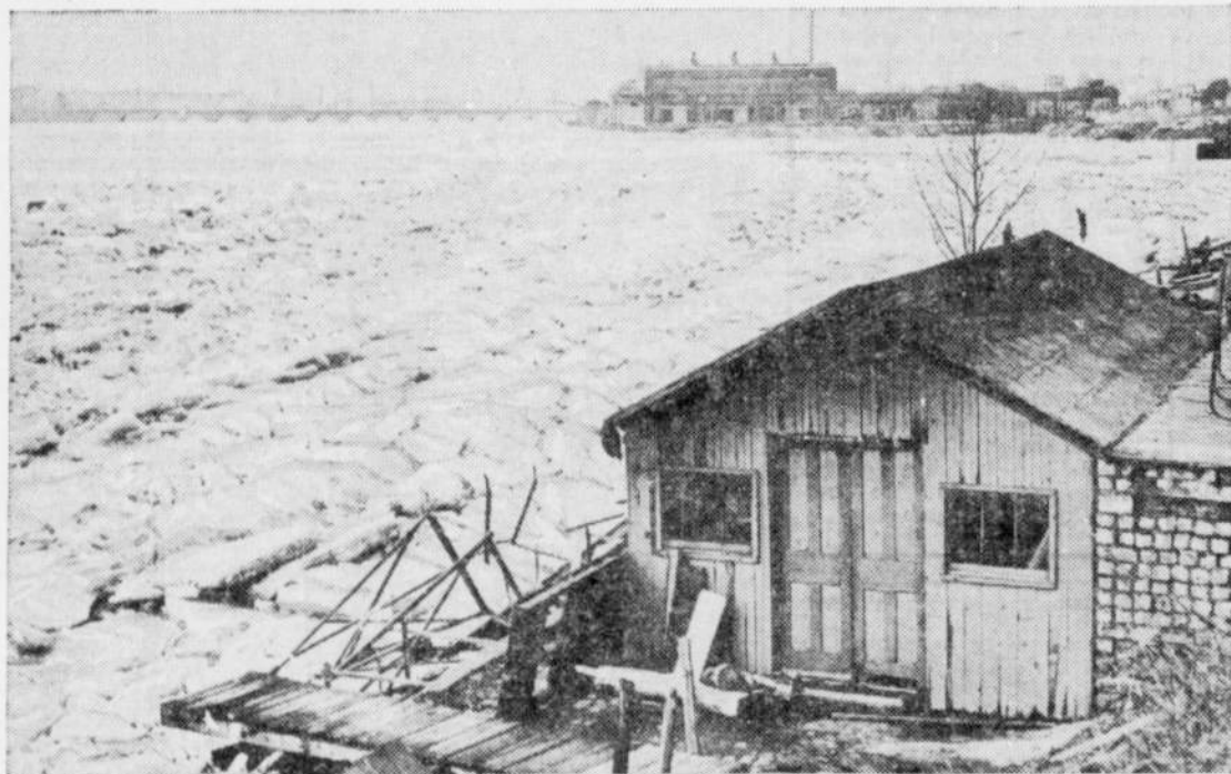
At its highest level in 31 years, the Delaware river's ice jam at Trenton, N. J., was at dangerous heights. It had overflowed a 12-foot retaining wall and flooded the municipal water plant, seen in the background, and many waterfront cellars. The huge ice cakes are shown being crunched against the shore.
