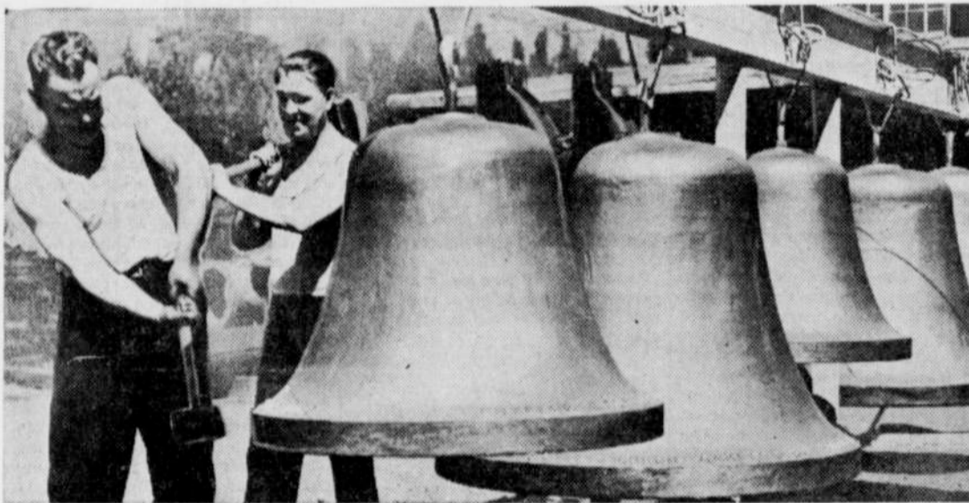
One of the many safety measures to be installed on the gigantic San Francisco-Oakland bay bridge is a group of five huge bells, one for each tower and the central anchorage. The bells, largest ever made in western America, have been undergoing tests in a San Francisco foundry for tone and carrying power. Workmen with sledge-hammers are seen pounding them. Each bell is of a different pitch and when installed they will resound over the bay like giant chimes.
