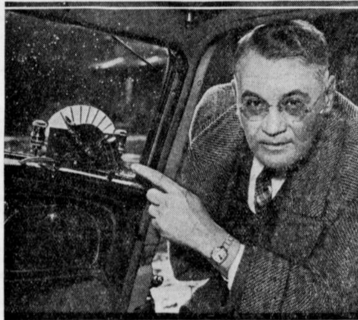
J. J. Huebscher of Minneapolis is shown with his regulating rheostat mounted on the cowl of a car just inside the windshield. The position of the dial determines the maximum speed of the car. A white light on the left burns at proper speeds, and a red light at right burns when the speed is excessive.
