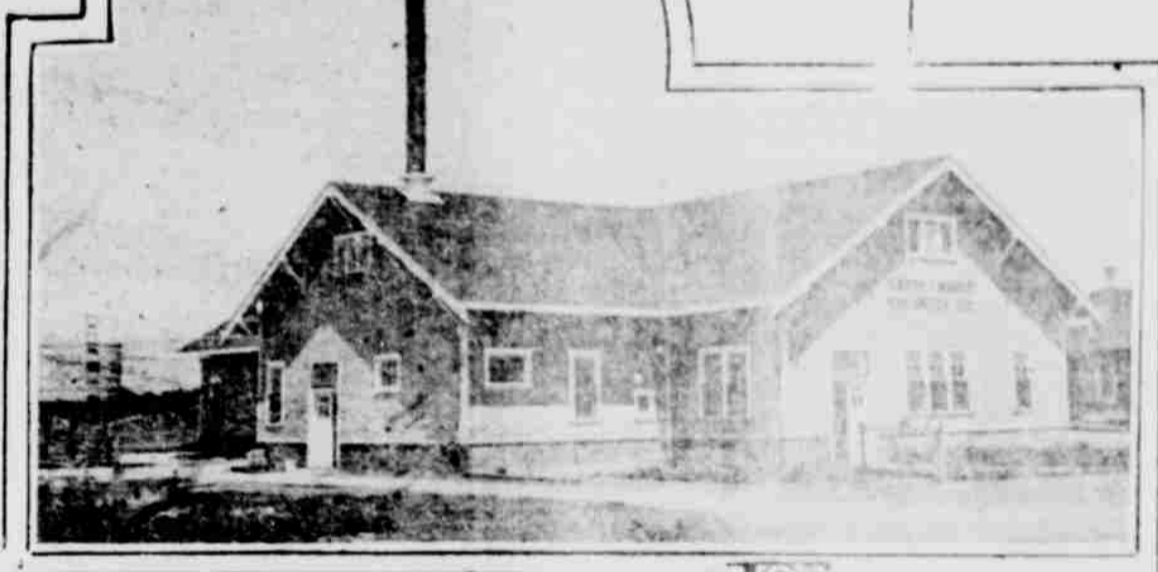
South Prairie Plant Recently Erected
