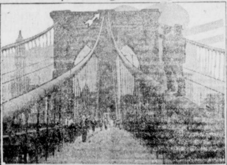
The largest suspension span on the famous old structure, the Brooklyn Bridge at New York, has slipped under the constant hammering of traffic and authorities have closed it to all except pedestrians...
