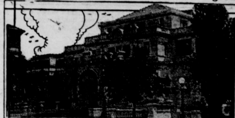
This structure is to be the official home of our vice-presidents, according to Washington reports. Vice-presidents have never been furnished with quarters. Mrs. Calvin Coolidge is said to have already inspected this home which is now nearing completion.
