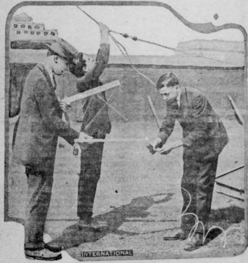
Amateur Radio Operators Erecting Aerial on the Roof.
