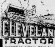
12 H. P. at the Draw Bar 20 H. P. at the Pulley High speed, heavy duty 4-cylender motor. 3 point spring suspen-sion. Weight 2750 lbs., height 52 inches, width 50 inches, length 96 inches, clearance 12 inches, 600 sq. inches traction surface.
