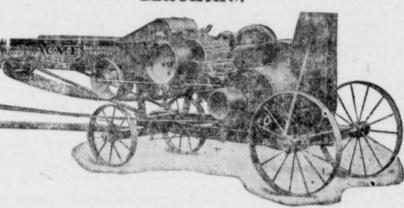
It has an all steel, Lowdown frame and steel truck. It has a malleable cutter head, malleable cutter bar, six fan blower, Alfalfa meal making attachment, and positive safety device, which marks an unusual not appear to be very susceptible, advance in the building of ensilege and feed cutting
