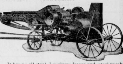
It has an all steel, Lowdown frame and steel truck. It has a malleable cutter head, malleable cutter bar, six fan blower, Alfalfa meal making attachment, and a positive safety device, which marks an unusual we may work upon the Sabbath, taken advantage of, however, in the advance in the building of ensilege and feed cutting machines
