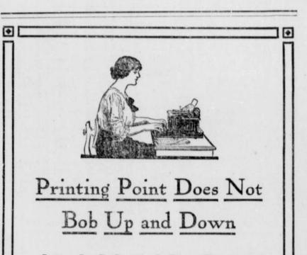
In an L. C. Smith & Bros. Typewriter the point on the paper which is to receive the type impression is stationary at the instant the type hits. The carriage does not bob up and down when the shift is made to write capitals.
