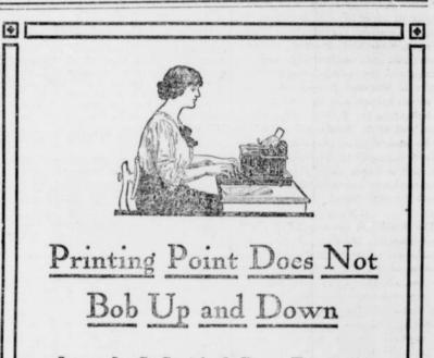
In an L. C. Smith & Bros. Typewriter the point on the paper which is to receive the type impression is stationary at the instant the type hits. The carriage does not bob up and down when the shift is made to write capitals. Why?
