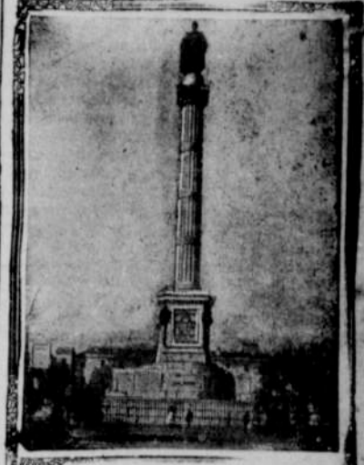
CALHOUN MONUMENT, CHARLESTON, S. C. covered with red ones. We went into St. Michael's church, one of the oldest churches in the South, twice injured by fire, and the walls cracked during the great earthquake. The three walls are lined with memorial tablets; the pews are of the old style, high ones,
