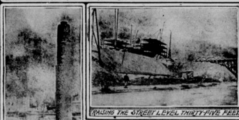
RAISING THE STREET LEVEL THIRTY-FIVE FEET. Views of NEW WASHINGTON R. R. STATION
